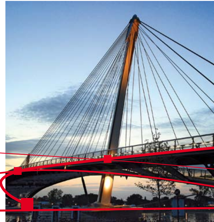
Cover picture: Passerelle des deux Rives between Kehl and Strasbourg (Stadt Kehl/Peter Heck)
